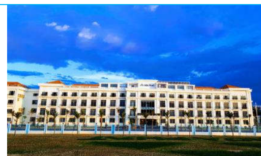
Project: Hoa Phat Dung Quat iron and steel factory Package: M&E system Client: HBC Value: 29.9 billion VND Time: 2017
