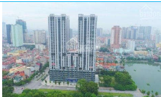
Project: HUD New Skyline Package: Electric Cabinet System Client: Technical JSC Value: 18 billion VND Time: 2016
