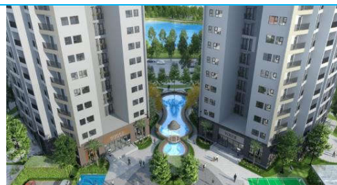
Project: BRG Package: M&E system for the basement Client: Hanco3 Value: 59.9 billion VND Time: 2020
