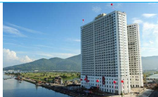
Project: Hoa Binh Green Da Nang Package: Air-conditioning and ventilation system Client: Hoa Binh Company Limited Value: 21.7 billion VND Time: 2017
