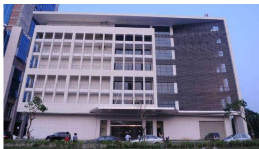
Project: Viettel Lang Hoa Lac General Data Center Package: Electric Cabinet System Client: Viettel IDC Value: 7.5 billion VND Time: 2016
