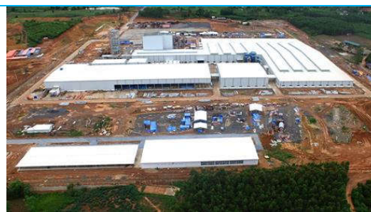
Project: Nghe An MDF Factory Package: Electric Cabinet System + Busway Client: Litech., Jsc Value: 23.3 billion VND Time: 2015
