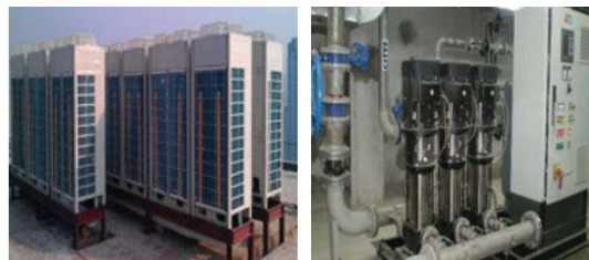
Project: FLC Vinh Thinh Resort Package: M&E system Client: Technical JSC Value: 22.1 billion VND Time: 2016
