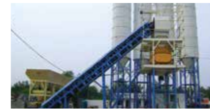
Trạm trộn bê tông 60m 3 Concrete mixing plant - capacity 60m 3
