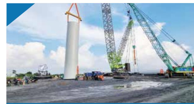
LẮP DỰNG TUABIN GIÓ/ WIND TURBINE ERECTION
